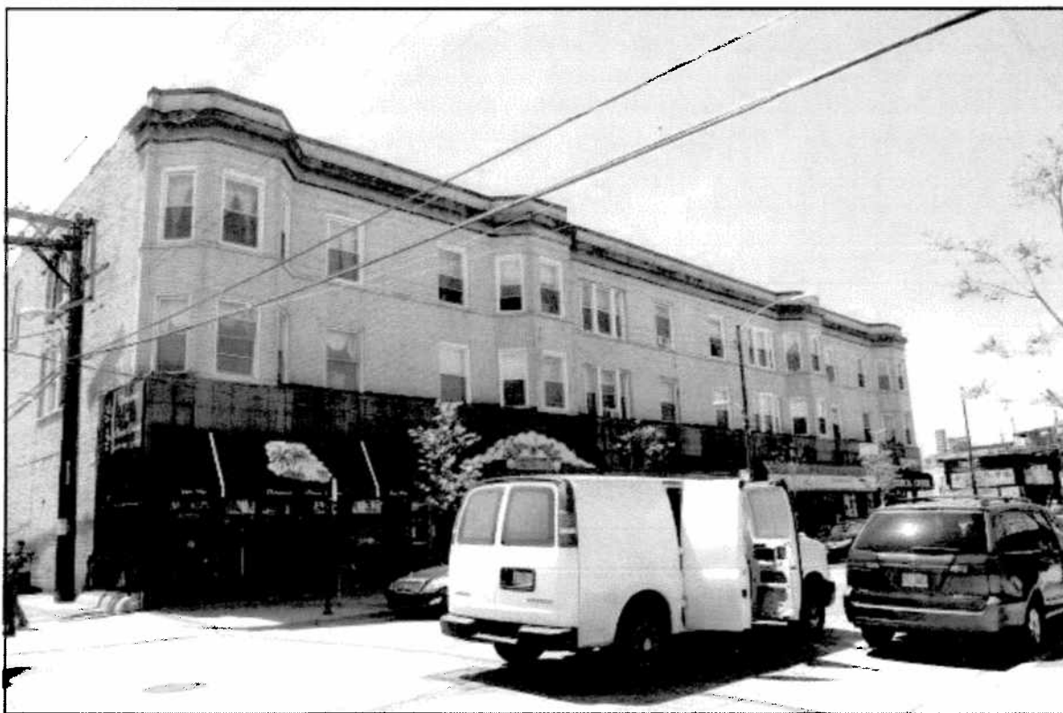
1055-1075 West Argyle Street (1908, with later storefront additions)
